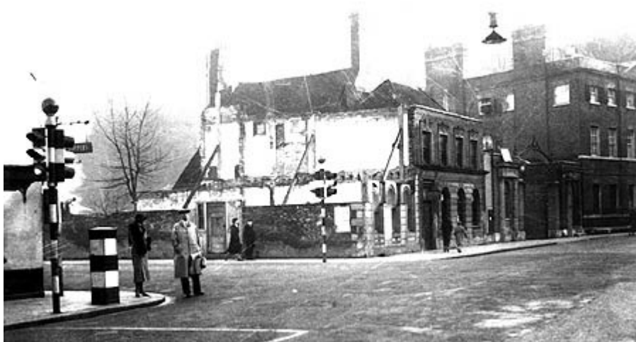
Demolition of The Windsor Brewery, circa 1933; © RWWS
